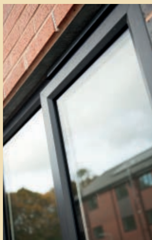
Bevelled profile frames in Anthracite Grey on the outside and white inside.
