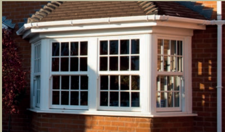
Bay window with vertical sliding Georgian bar sash windows.
